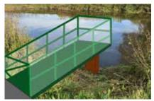
Langport flow station Ground investigations were completed and a flow gauge station was designed. The data it collects (after construction in 2021) will help to improve flood risk management across nearly 500 square miles.
