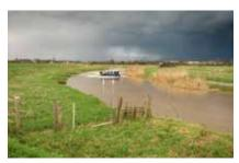
**River Parrett pioneer dredging** Dredging of 1.37 miles of the River Parrett down to the M5 bridge removed around 22,000m<sup>3</sup> of consolidated silt deposits. Dredging is combined with a sophisticated programme of silt monitoring.
